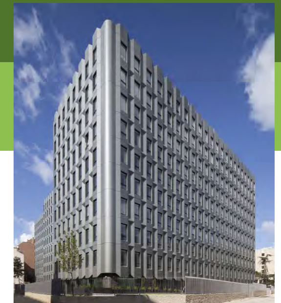
Chevaleret à Paris, France NF HQE™ Certificat Excellent & BREEAM® Certificat Very Good ALUCOBOND® Grey Metallic Architectes Archigroup (renovation) / Novarina © Milène Servelle
