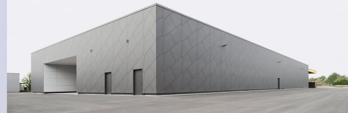
Supply shed in Niederstetten, Germany (A+D 56, p. 20)
