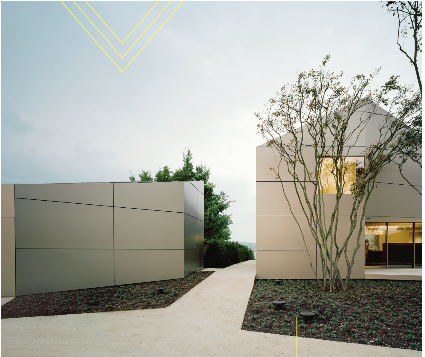
Villa at Lake of Constance, Germany Biehler Weith Associated ALUCOBOND® PLUS anodized look C32 © Brigida González
